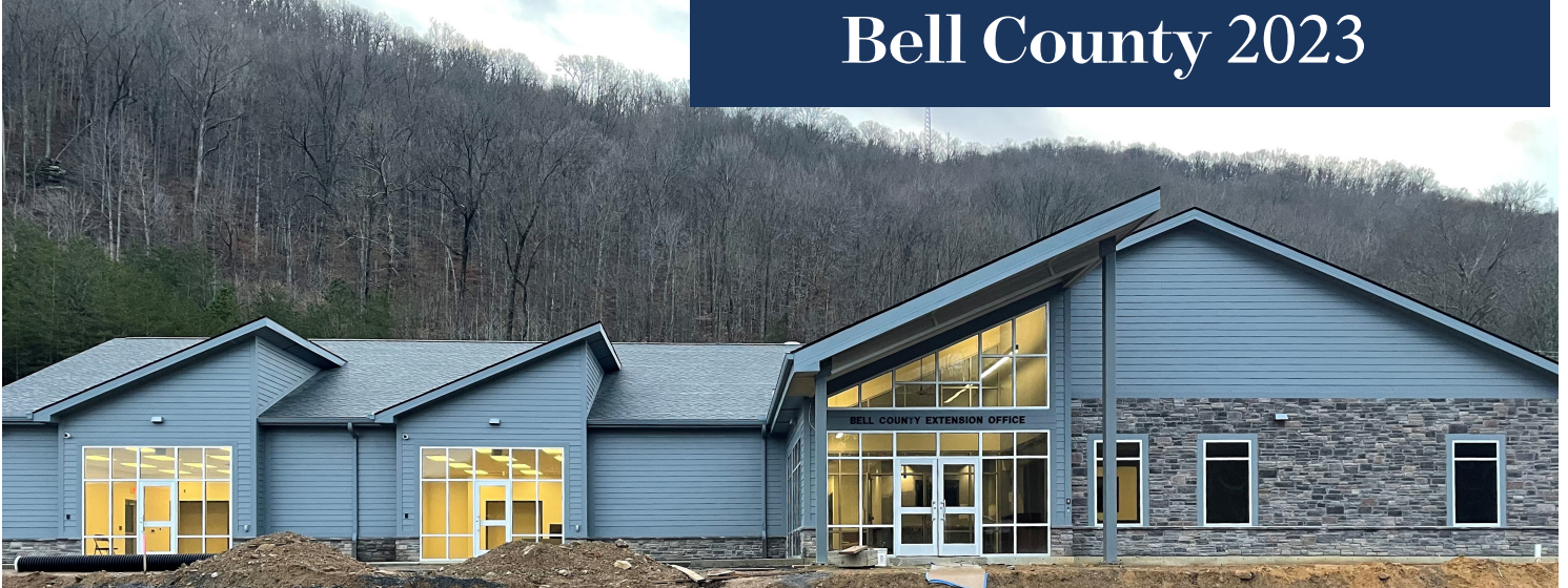
Bell County Extension new building under construction
